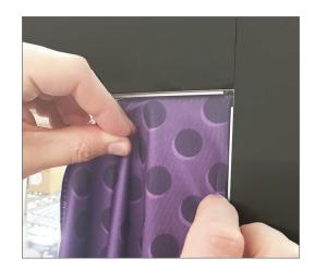
1 Starting with the top right hand corner of the frame, insert about an inch of the silicone gasket into the metal track. Repeat this process on the top left and bottom corners.
