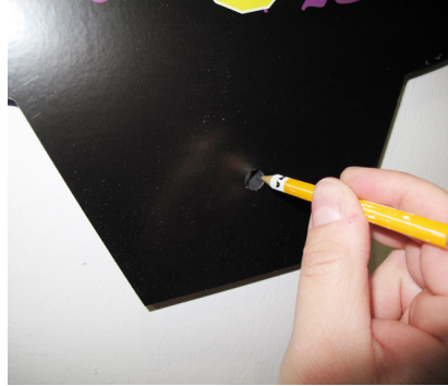
2 Place sign on the wall to mark the holes for the standoffs.
