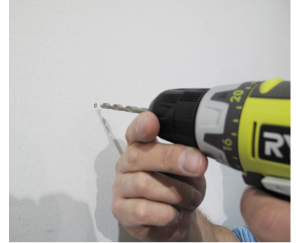
3 Drill pilot holes (use anchors, if needed).
